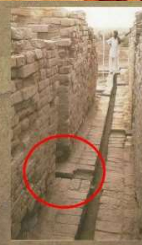
Drains in houses connected to those on streets
