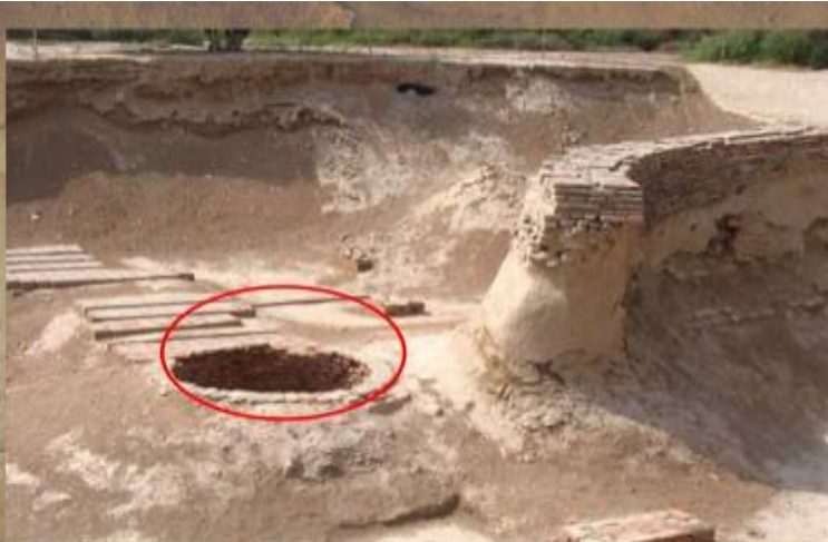
Inspection holes for closed drains
